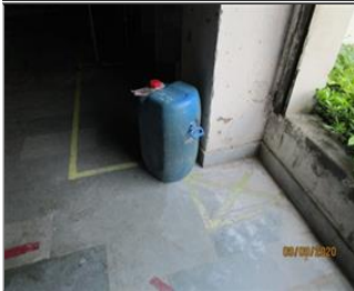
Photo of non-conformity secondary containment was not provided to diesel drum.JPG
