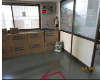
Photo of non-conformity fire extinguisher was found blocked.JPG
