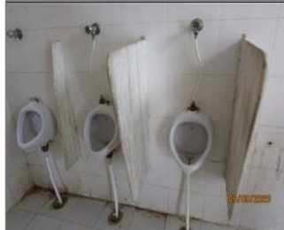
Photo of the sanitary facilities toilet 02.JPG
