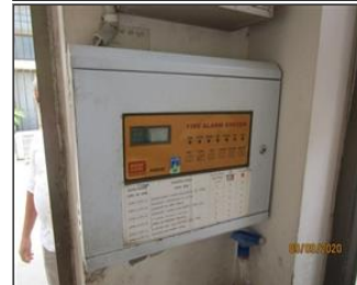
Photo of fire safety equipment fire panel.JPG
