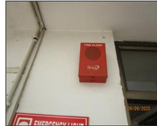
Photo of fire safety equipment fire alarm.JPG
