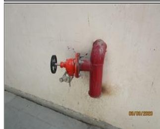
Photo of fire safety equipment hydrant.JPG
