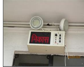
Photo of fire safety equipment emergency light.JPG
