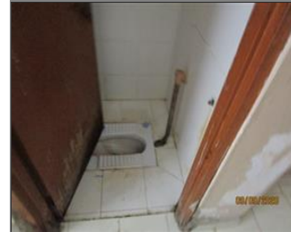
Photo of the sanitary facilities toilet 03.JPG
