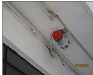
Photo of fire safety equipment fire hooter.JPG
