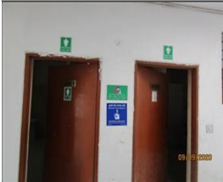
Photo of the sanitary facilities toilet 01.JPG
