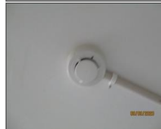
Photo of fire safety equipment smoke detector.JPG
