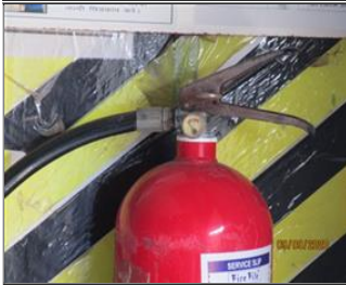
Photo of non-conformity low pressure was found in fire extinguisher.JPG
