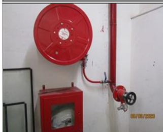
Photo of fire safety equipment hose reel and hydrant.JPG
