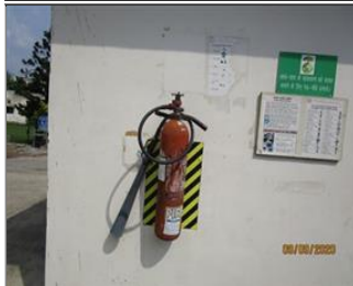
Photo of fire safety equipment fire extinguisher.JPG
