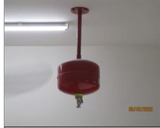
Photo of fire safety equipment ceiling mounted fire extinguisher.JPG
